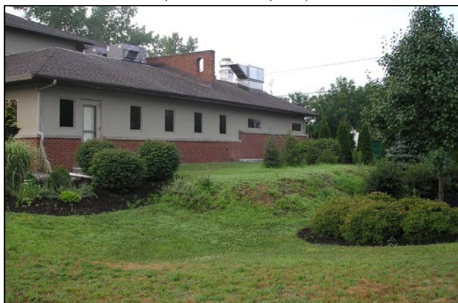
Figure 5.38 Rooftop disconnection for storage and infiltration, Guilderland, NY, NYSDEC
