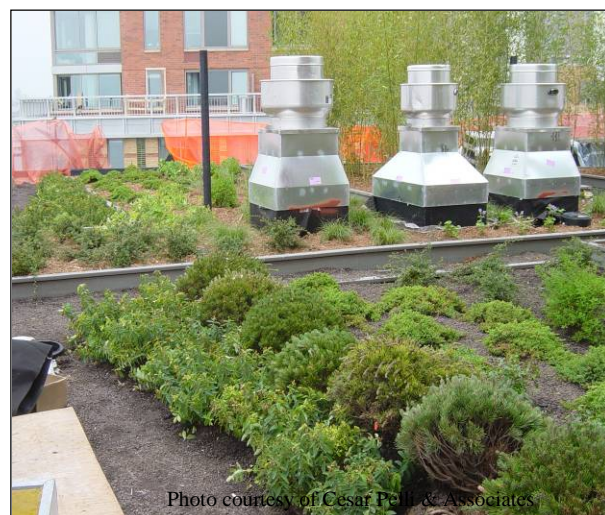
Figure 5.46 Green roof on a Manhattan apartment building along the Hudson River
