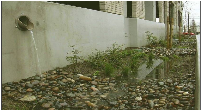
Figure 5.54 This flow-through planter collects runoff from the rooftop of a parking garage and is incorporated into the structure
