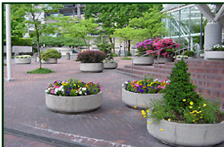
Figure 5.53 Contained stormwater planters made of concrete
