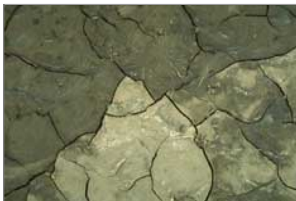
Figure 5.14 Shows typical compacted soils that nearly reach the bulk density of concrete (Schueler et al 2000)
